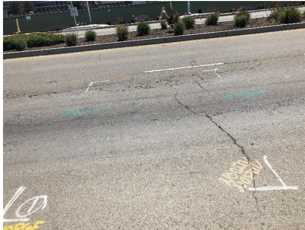
FIGURE 1: Transverse Cracking
