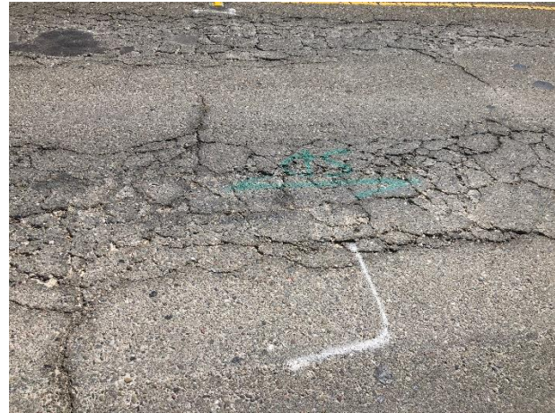
FIGURE 2: Alligator Cracking
