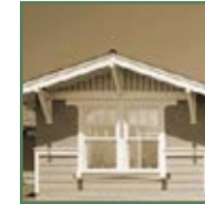
Decorative gable-end detailing
