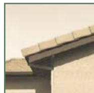
Chamfered rafter tails
