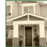
Decorative gable-end portal
