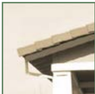
Square rafter tails
