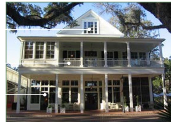
Single hung windows with mullions
