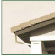
Square rafter tails
