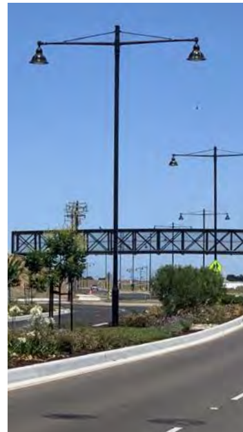
Arterial Street Lights
