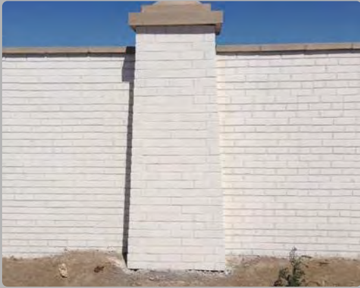
8' Tall Masonry Column with 6' Tall Community Masonry Wall
