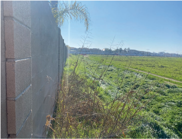
PHOTO 1: MOSSDALE LANDING WEST ALONG EASTERLY WALL
