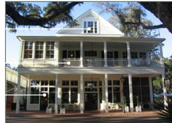
Single hung windows with mullions
