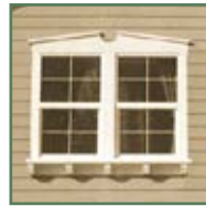
Sill with corbels
