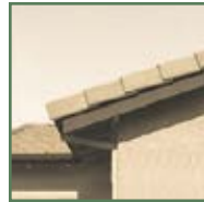
Chamfered rafter tails
