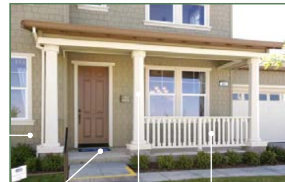
Entry Porch Square columns Pickets
