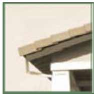
Square rafter tails
