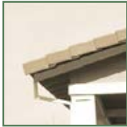
Square rafter tails
