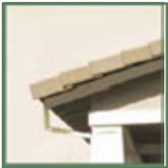
Square rafter tails
