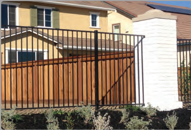
8' Tall Masonry Column with Open View Fence (5' Tubular Steel Fence @ Linear Park & Lake Frontage)
