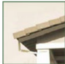
Square rafter tails
