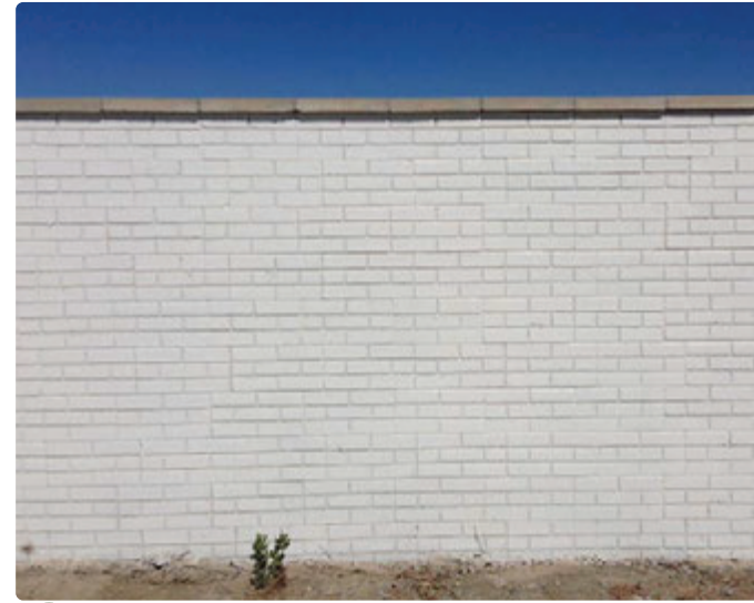
6' Community Masonry Wall
