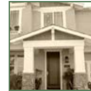
Decorative gable-end portal
