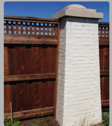
8' Tall Masonry Column with Decorative Wood Community Fence
