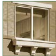
Sill with corbels
