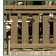
Cut out panels
