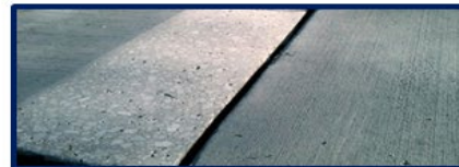
ADA Compliant Trip Hazard Repair
