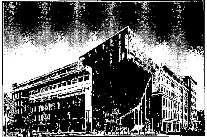
San Joaquin County Administrative Building
