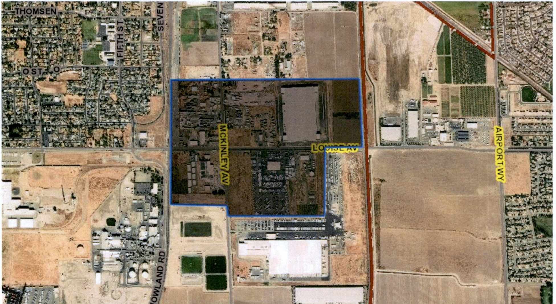
Note: Extent of Parcels Used to convey Flows to McKinley Sewer Pump Station via E. Louise Avenue and McKinley Avenue Gravity Sewer Main
