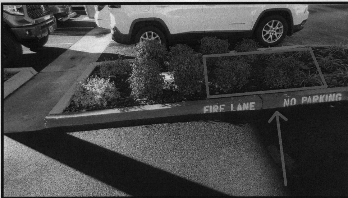
Additional Image of the South-East Side of the Lathrop City Hall Parking Lot.
